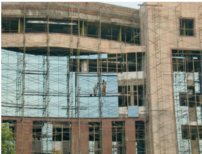
Typical commercial building with sandstone cladding, under construction in Gurgaon around 2003.
