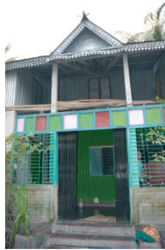
The 'height factor' in Sharifa's two-storeyed bungalow is less about a real need for space than about the family's yearning for social visibility. Although an elevated verandah overlooks the surrounding landscape, the first floor is used mostly for storage.
