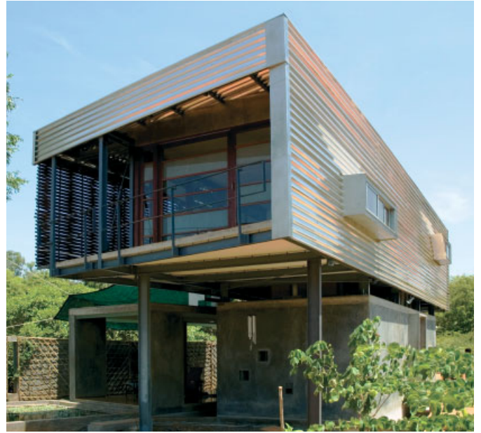
Fabian Ostner, House for Klara, Auroville, 2003 A hybrid and structurally challenging building, this house attempts to create interesting and aesthetic living spaces within a flexible steel structure using industrial materials not commonly found in India's residential architecture.
