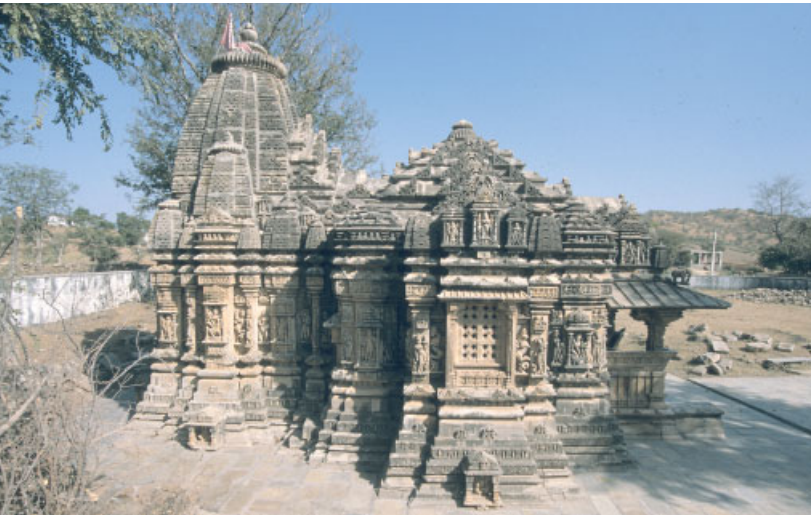
The Ambika Temple, Jagat, from the south. A porch leads to the mandapa , audience hall of the enshrined deity, leading via an antechamber to the dark sanctum beneath the tower. Above the antechamber, divine power is radiated from the front of the tower through a cascade of pullulating horseshoe arch dormer motifs ( gavakshas ).
