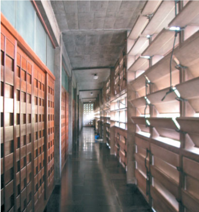
Antonin Raymond, Golconde, Pondicherry, Tamil Nadu, 1945 India's first example of Modern architecture and of the first use of reinforced cement concrete commissioned by the founders of Auroville, continues to serve as a bench mark for the high standard of architecture aspired to at the time. The building still stands as one of the best examples of climatic comfort through passive cooling, its entire facade composed of custom-made prefabricated operable asbestos louvres to let in the southeast breeze.
