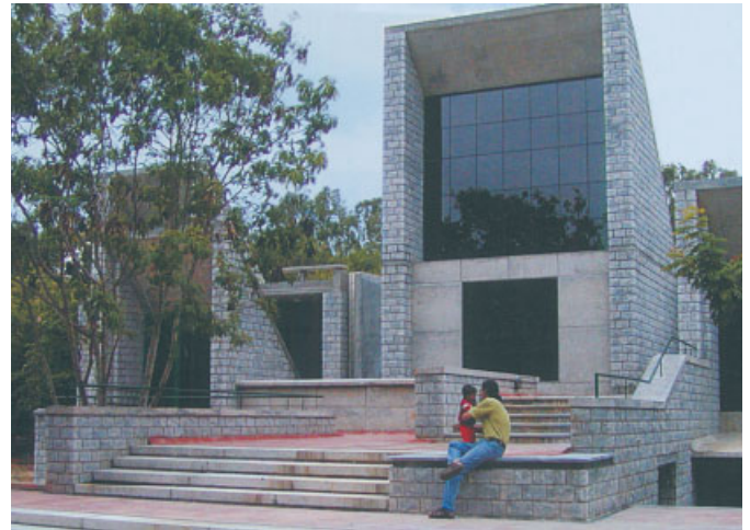
Sanjay Mohe, GIV Building, Bangalore, 2003 Locally quarried grey granite is used in both the original complex and in this recent addition to the Balkrishna V Doshi Indian Institute of Management of 1985.
