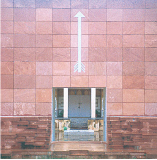
Charles Correa, Jawahar Kala Kendra, Jaipur, 1992 Another example of the use of local red sandstone.
