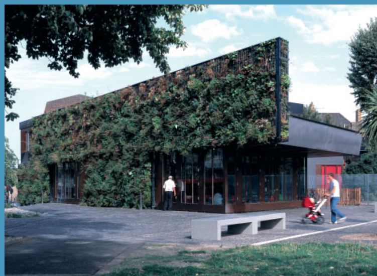
Paradise Park Children's Centre and Park Café, Islington, London, 2006 A Sure Start initiative, this nursery, café and training facility was part of the regeneration of a run-down park in North London. Its key feature is the vertical hydroponic garden covering the front elevation, an innovative response to planning policy that asked for green spaces not to be lost.
